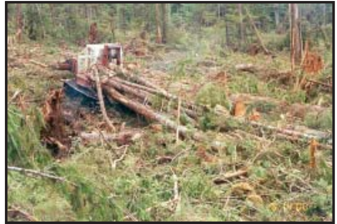
Figure 5. FMC tracked skidder moving logs to the landing.
